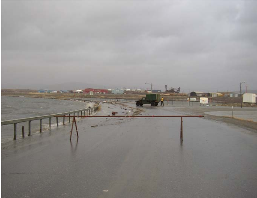
Photo 1: Storm surge on Seppala Drive looking north away from Harbor towards the airport; photo courtesy of City of Nome, October 2004.
